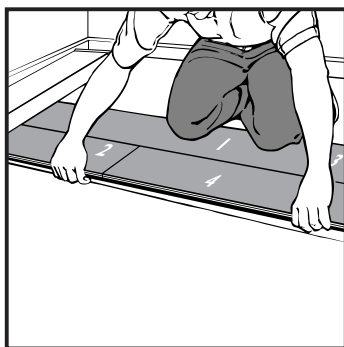
[10] Place hand under locked ends of 2 and 4, raise slightly, pull plank 4 into plank 3 edge groove. Snap assembled group down into place.
